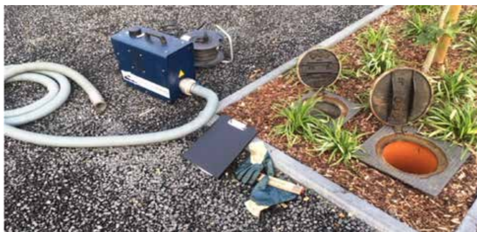
Picture 1: Testing of private sewer connections
